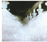
发电厂脱硫塔喷淋
